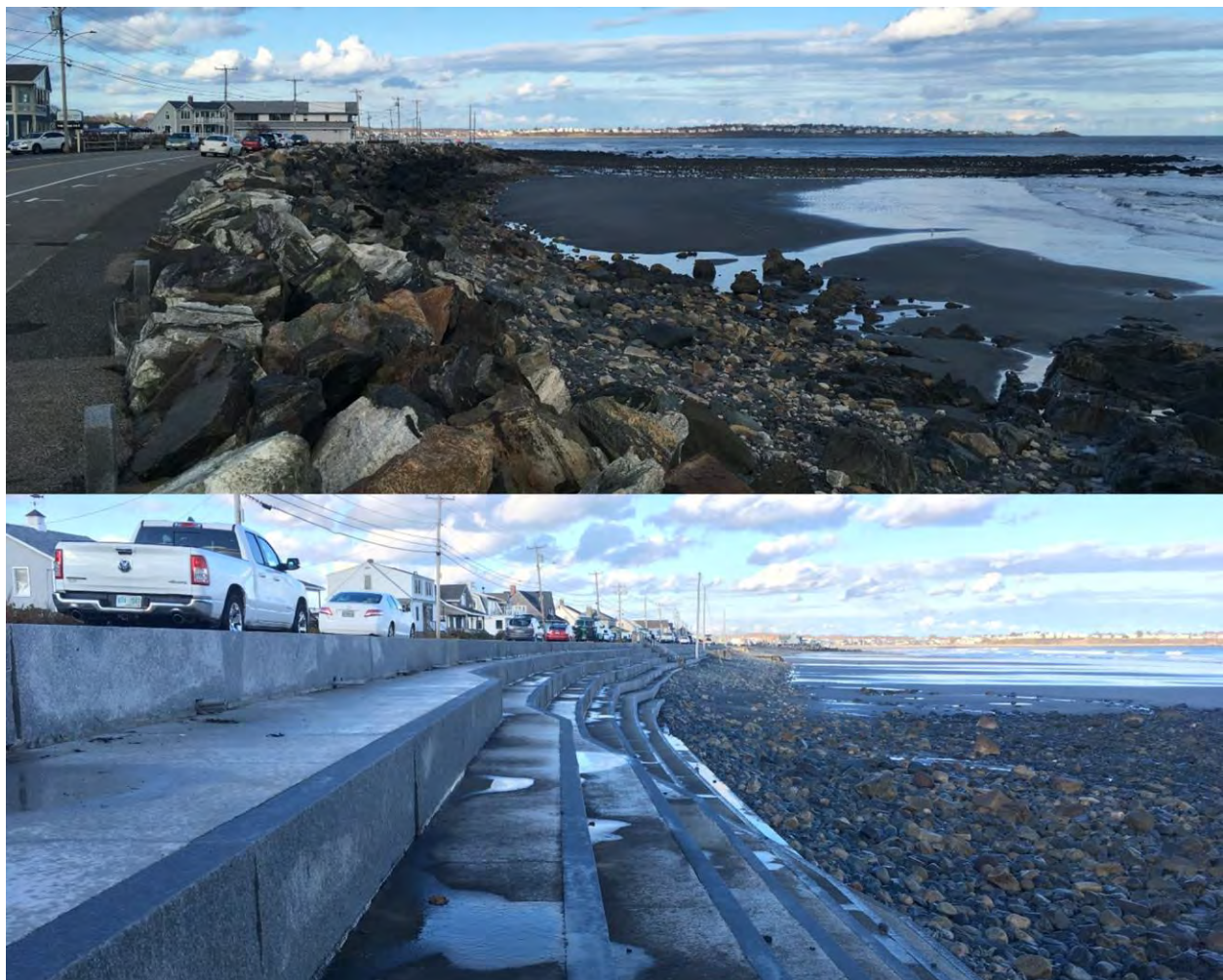
Examples of rip-rap (top) and seawall (bottom) along Long Sands Beach.
